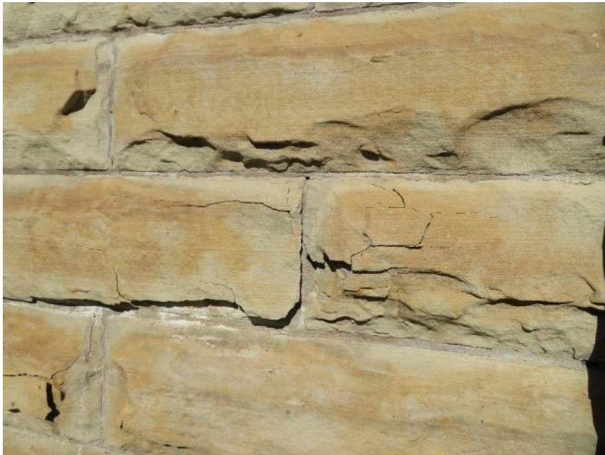
Spalling sandstone
