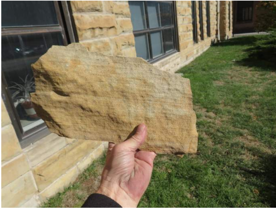
Spalled sandstone
