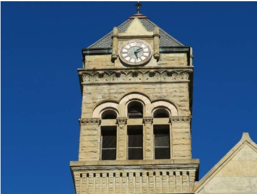
South Elevation of Clock Tower
