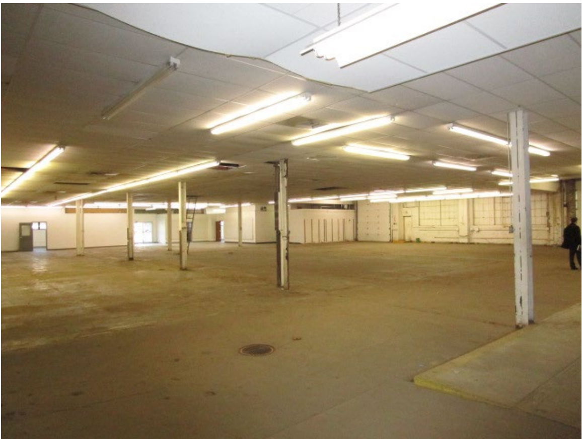
Photo #18. Main floor looking NE, shot 01-08-19.
