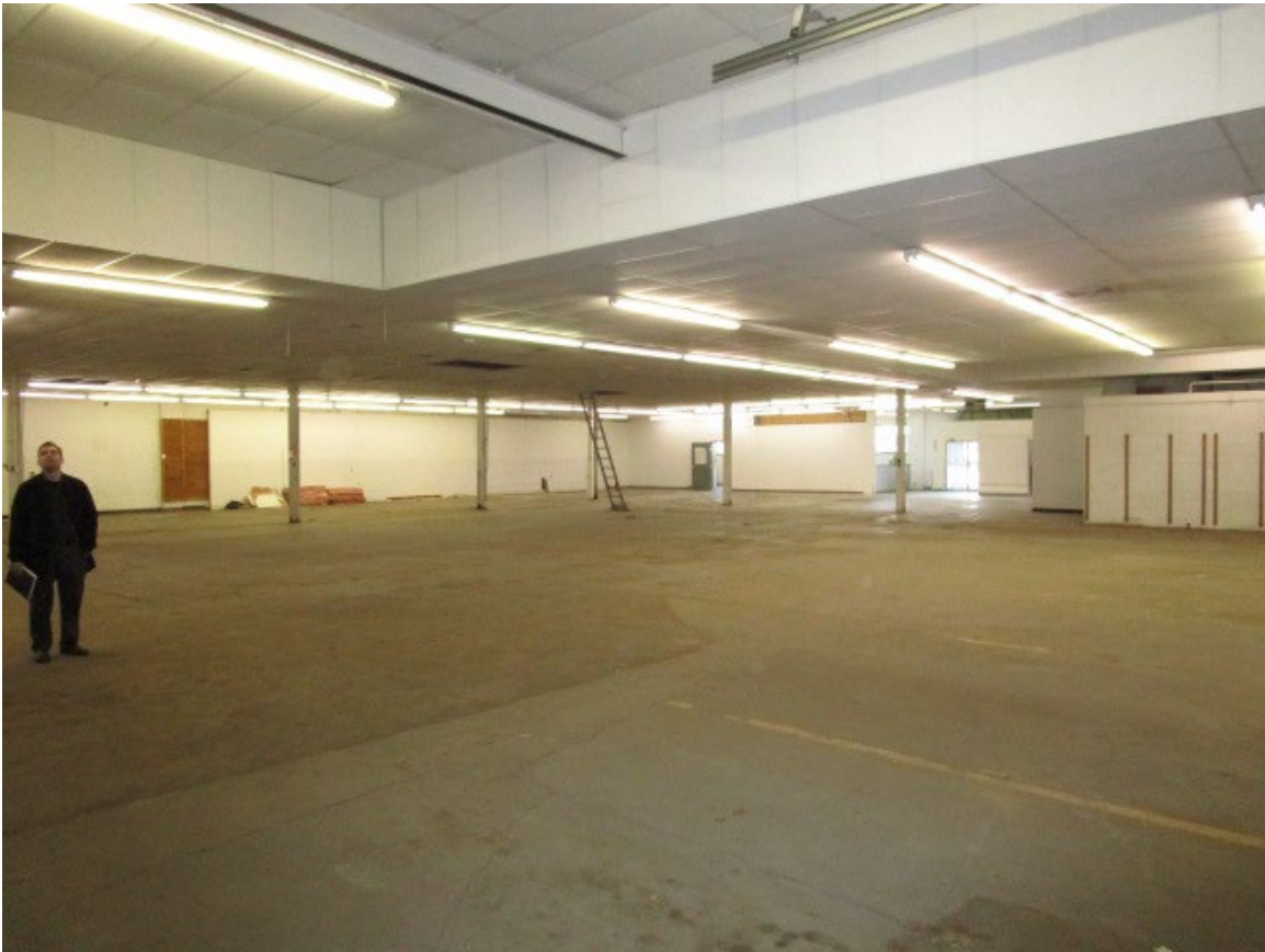
Photo #19. Main floor looking NW, shot 01-08-19.
