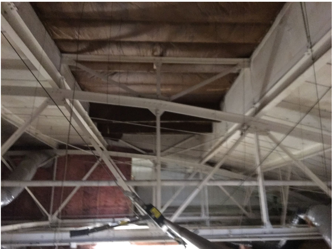
Photo #23. Bowstring trusses exposed looking N, shot 01-08-19.
