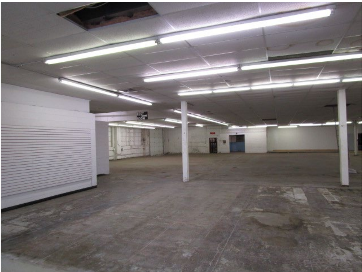
Photo #16. Main floor looking SSE, shot 01-08-19.
