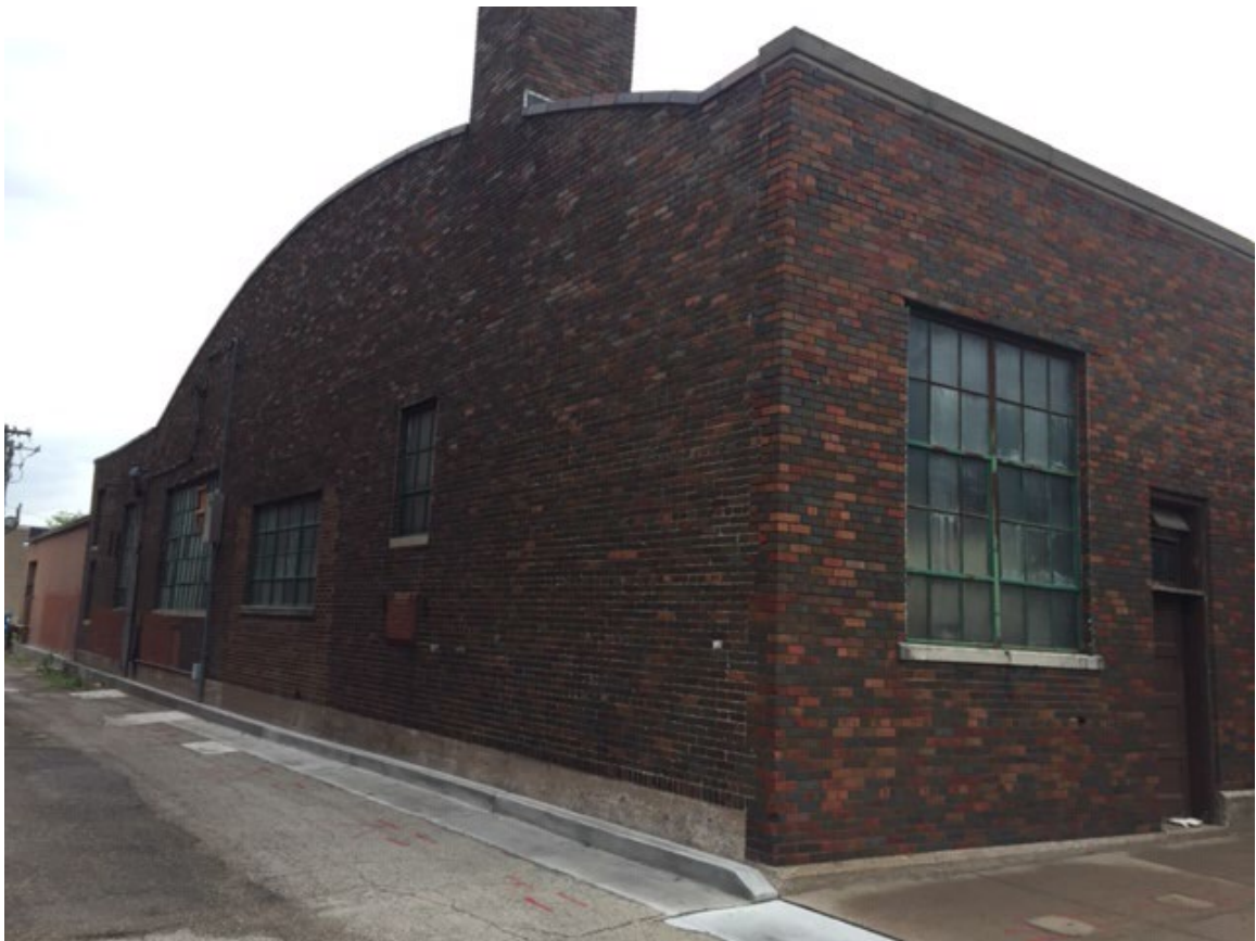
Photo #6. South elevation (left) & east elevation (right) looking NW, shot 05-15-22.
