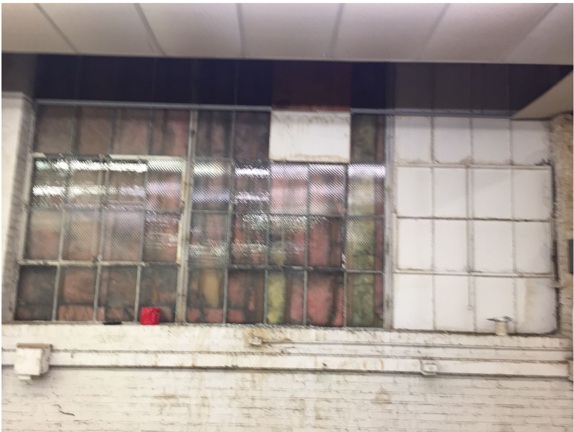
Photo #20. Typical commercial style window looking E, shot 04-14-20.
