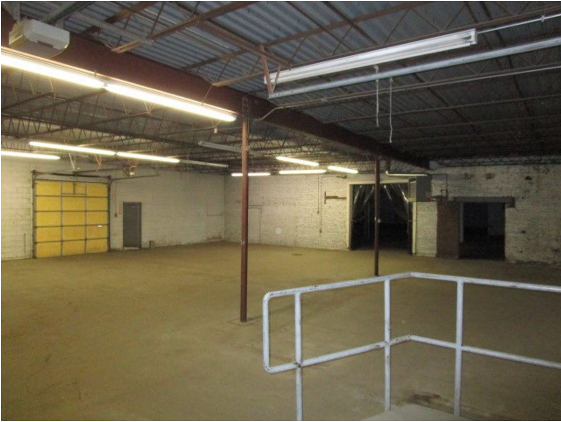
Photo #24. Addition looking NE, shot 01-08-19.
