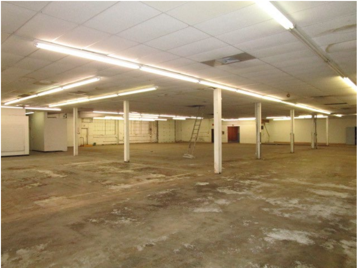
Photo #17. Main floor looking SE, shot 01-08-19.
