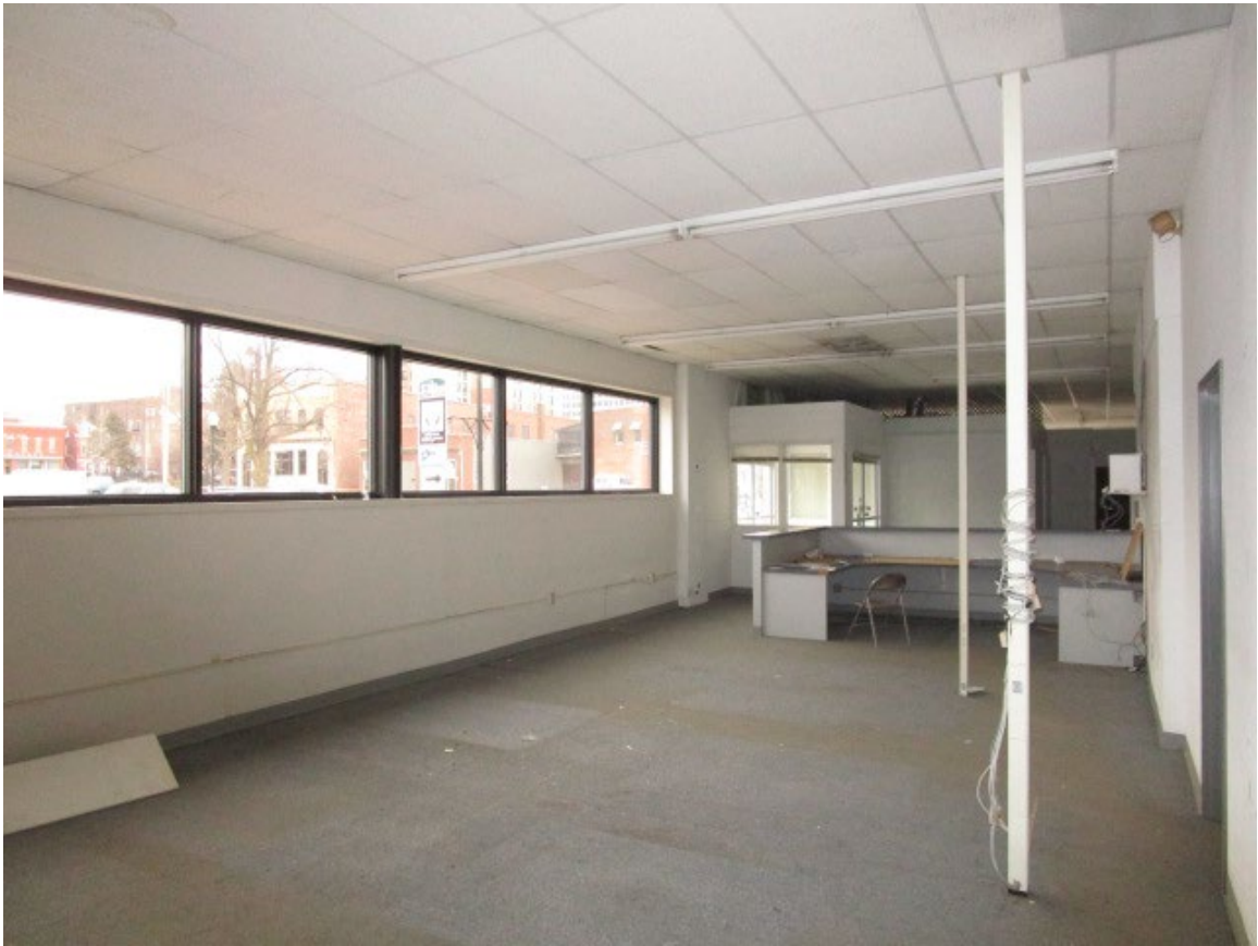
Photo #13. Main office w/entrance vestibule (center) looking NE, shot 01-08-19.
