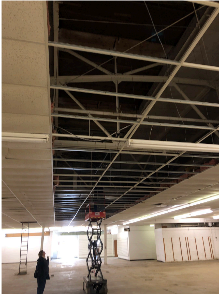
Photo #21. Roof trusses exposed looking N, shot 01-08-19.
