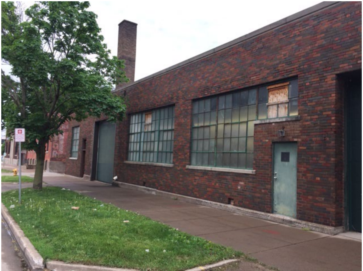
Photo #5. East elevation (south side) looking SW, shot 05-15-22.
