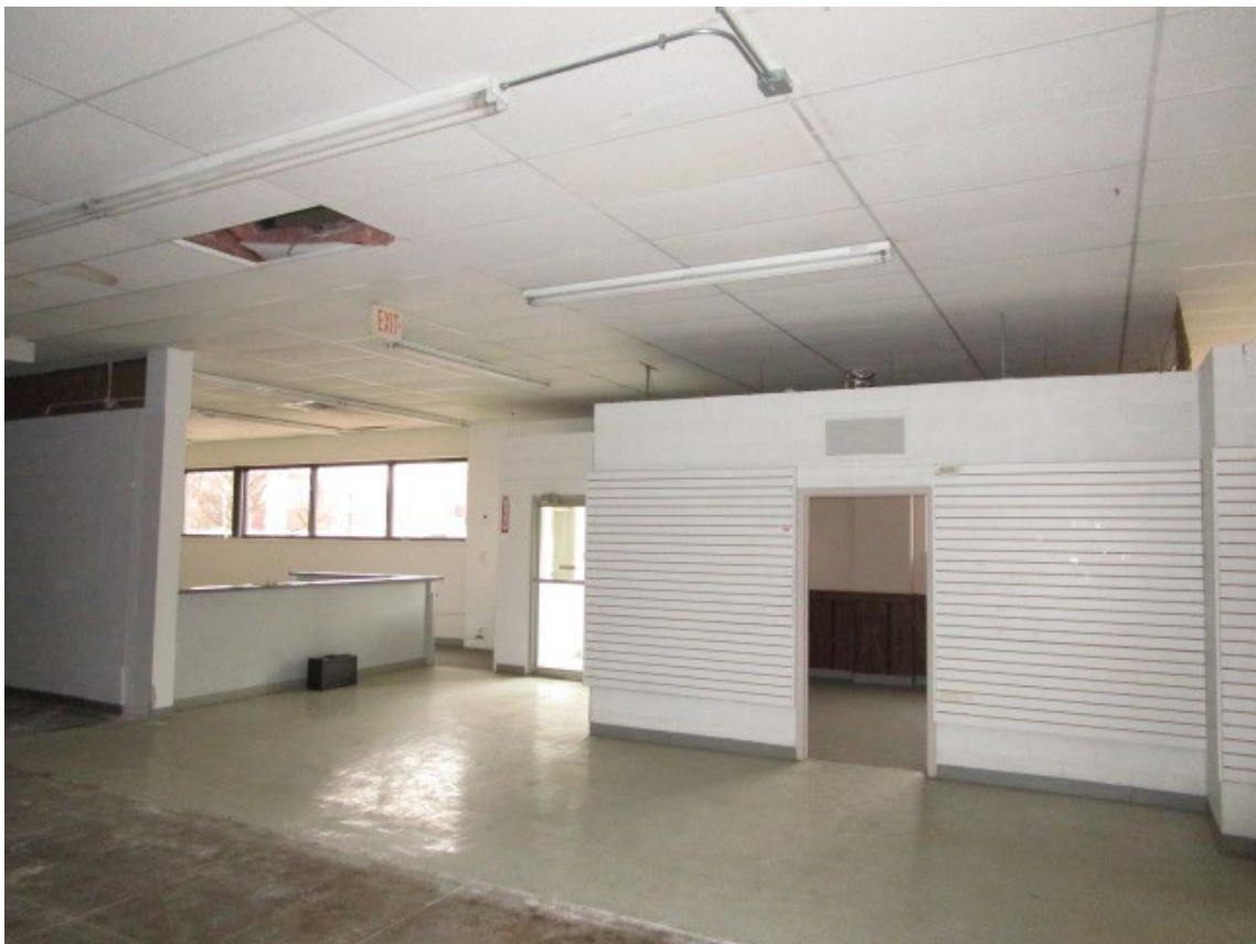
Photo #12. Lobby w/entrance vestibule (center left) looking NW, shot 01-08-19.
