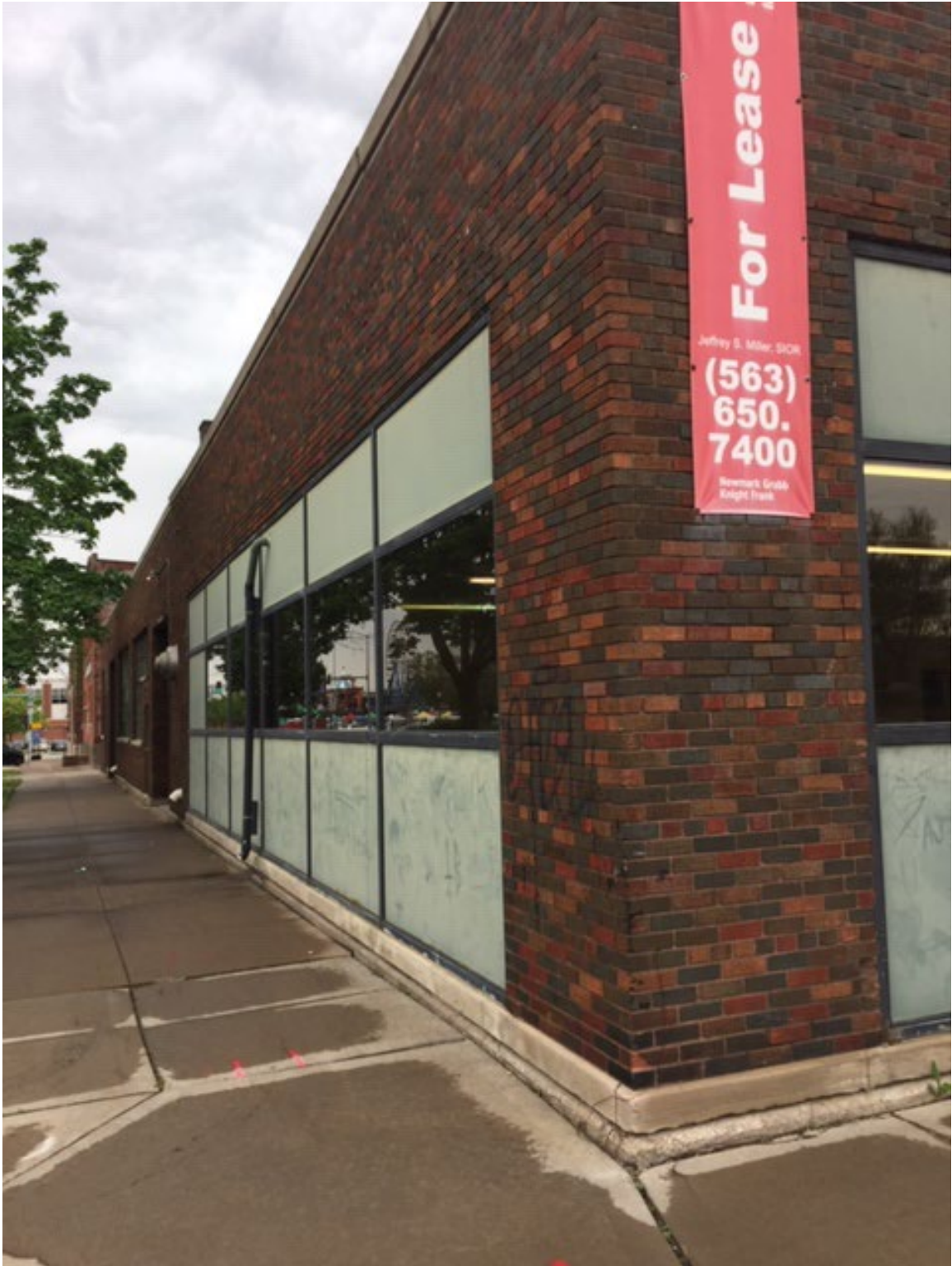
Photo #4. East elevation (north side) looking SW, shot 05-15-22.
