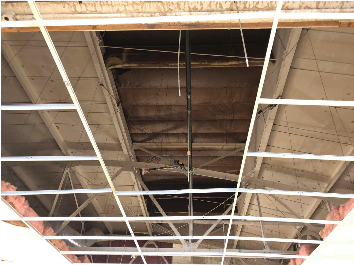
Photo #22. Skylight exposed looking N, shot 01-08-19.
