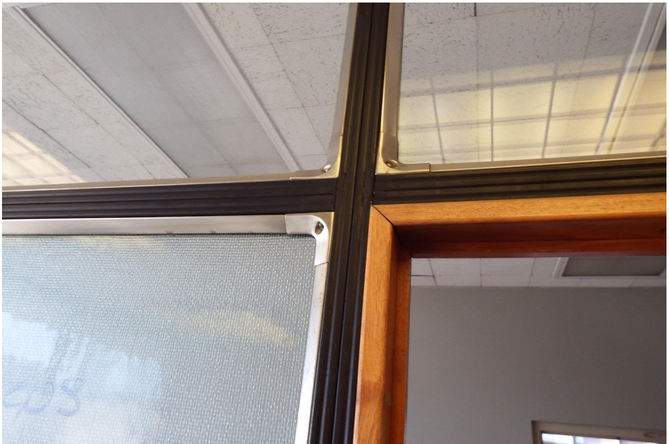
Photo 19: Interior, second floor, metal/glass demising partition detail, manager's office, looking west
