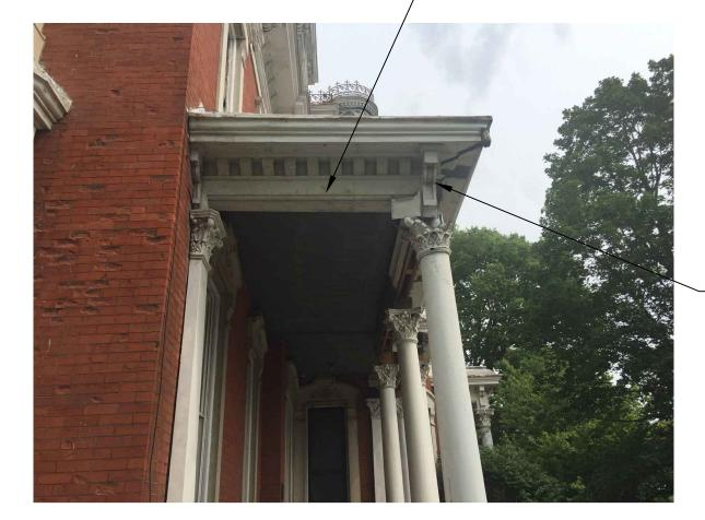
RELOCATE DAMAGED -CAPITAL TO LESS NOTICEABLE LOCATION AT OPPOSITE END OF RAILING & REPLACE WITH CAPITAL IN GOOD CONDITION
