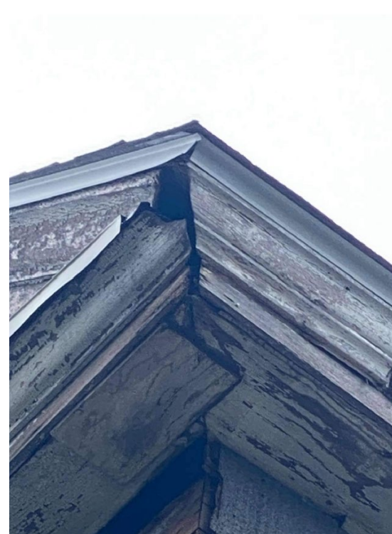
Deteriorated Wood Fascia & Soffit
