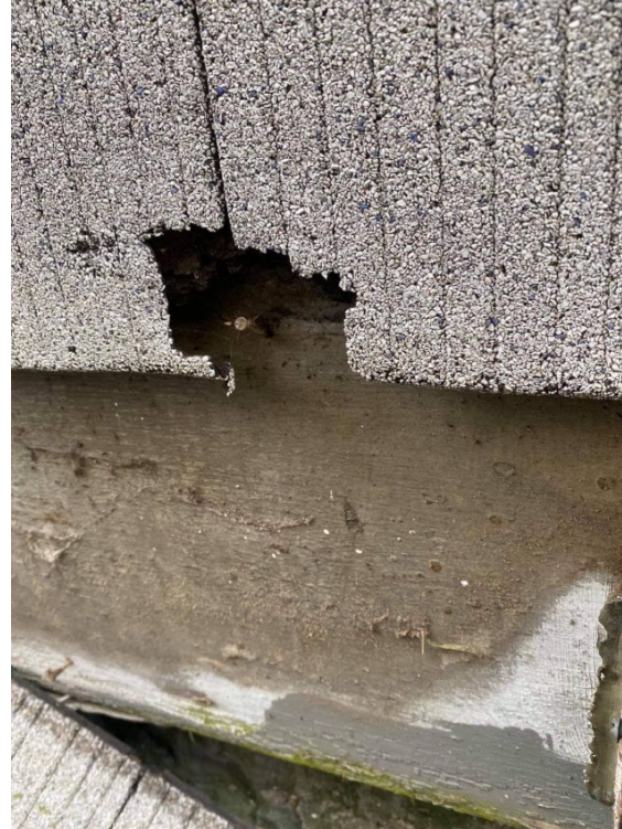
Deteriorated Wood Fascia & Soffit
