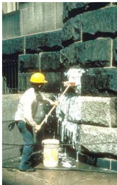
Chemical cleaning to remove dirt from granite.
