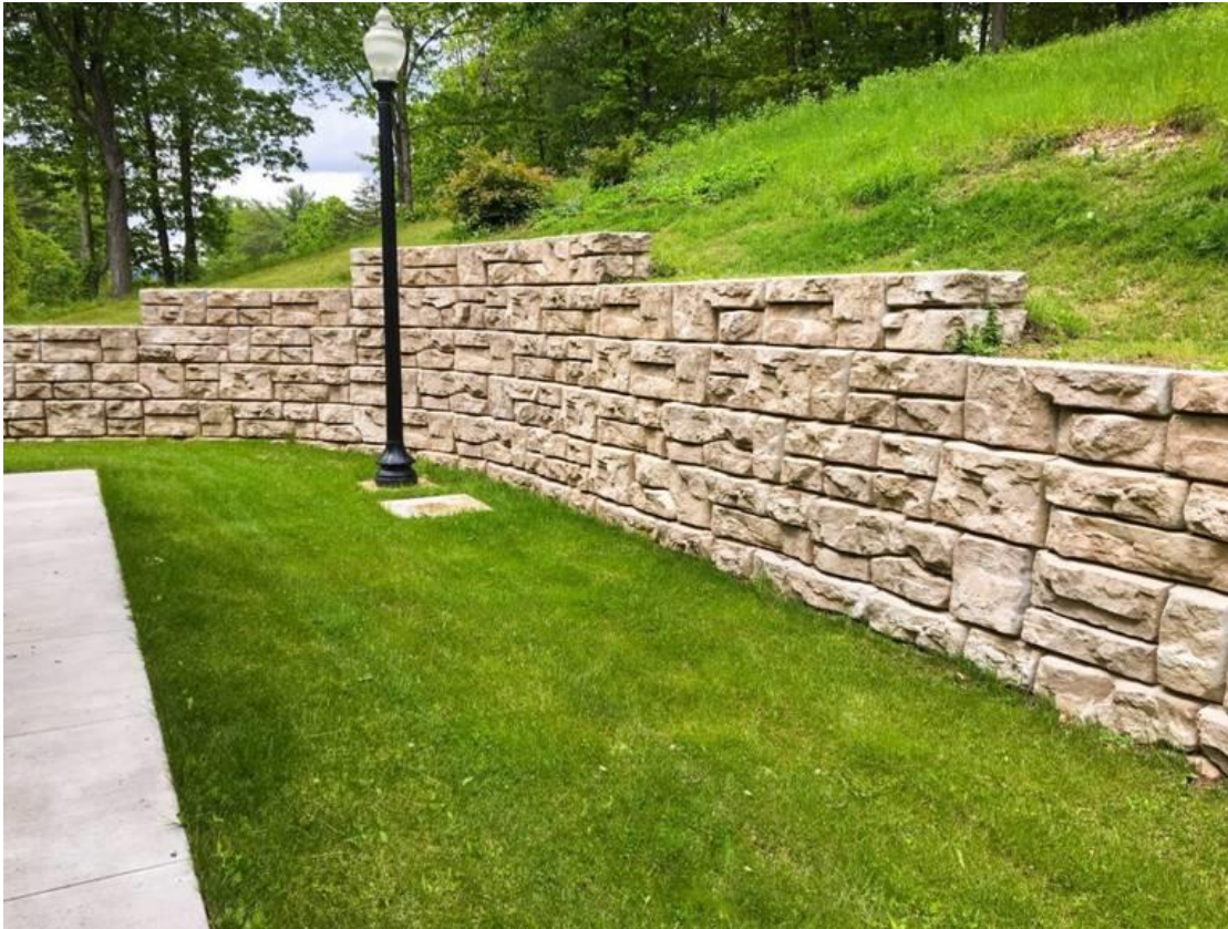
Replacement Redi-Rock Stone Ledgestone Option w/ Concrete Stain
