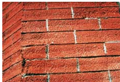
Historic brick damaged by sandblasting.
