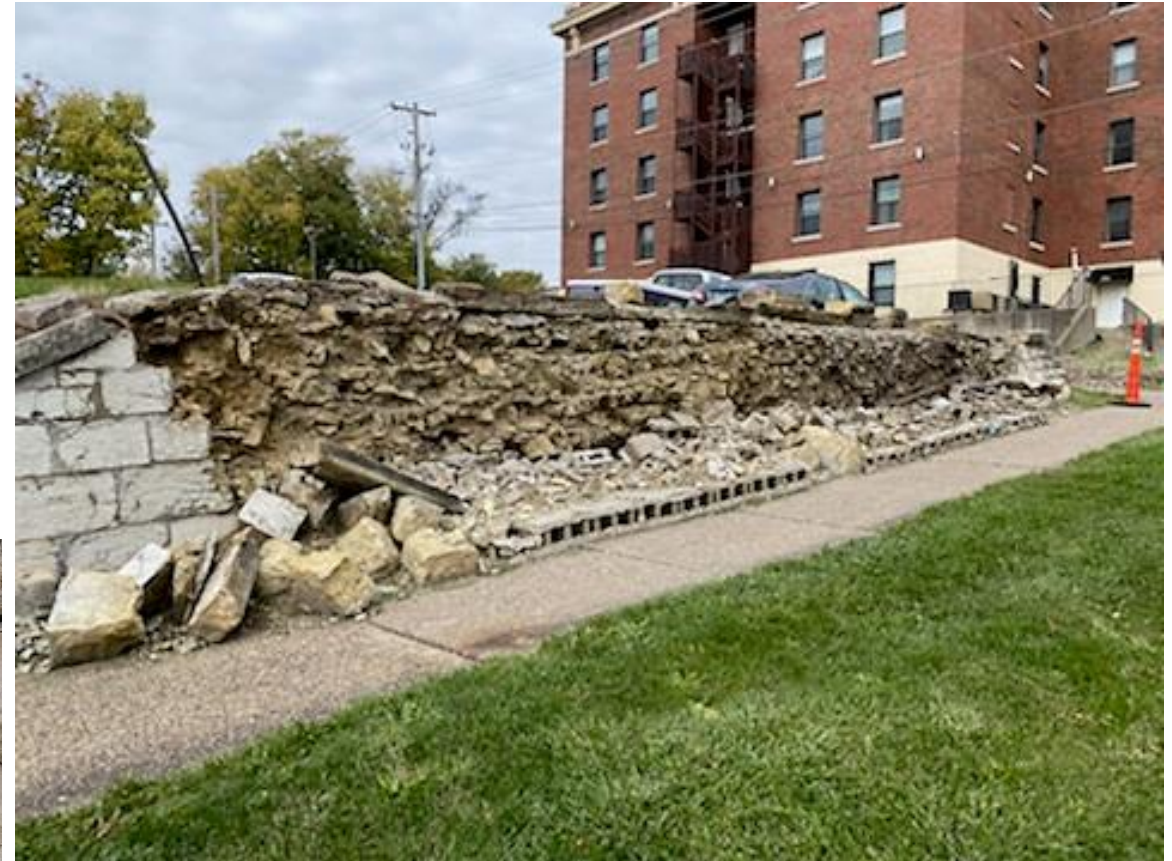
Example: Failed Retaining Wall at East 6 th Street & Iowa Street
