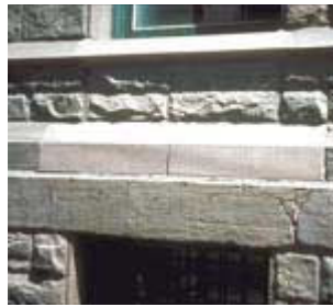
Replacement stones tooled to match original.
