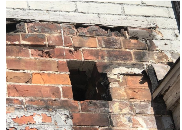
Missing Brick at Rear Elevation
