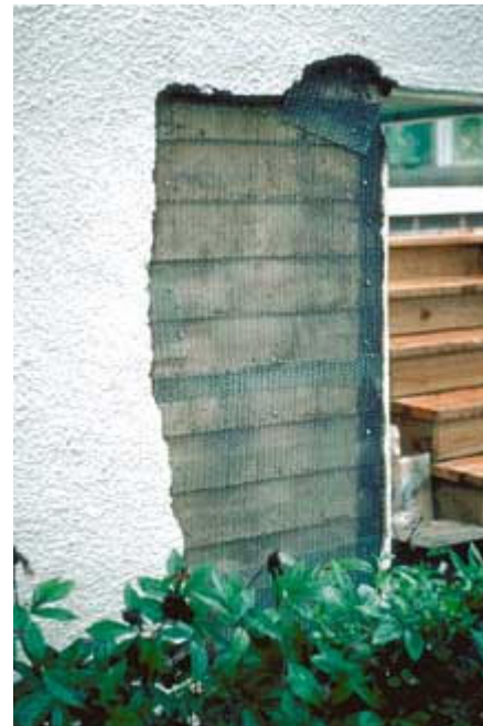
Preparation for stucco repair.
