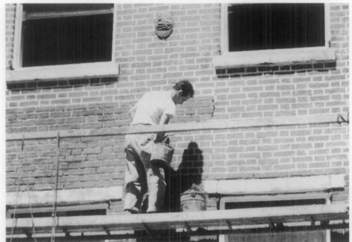
Figure 17. This photograph shows the significant visual change to the character of this historic brick building that has resulted from improper repointing procedures and a noticeably increased thickness of the mortar joints. Photo: Lee H. Nelson, FAIA.
