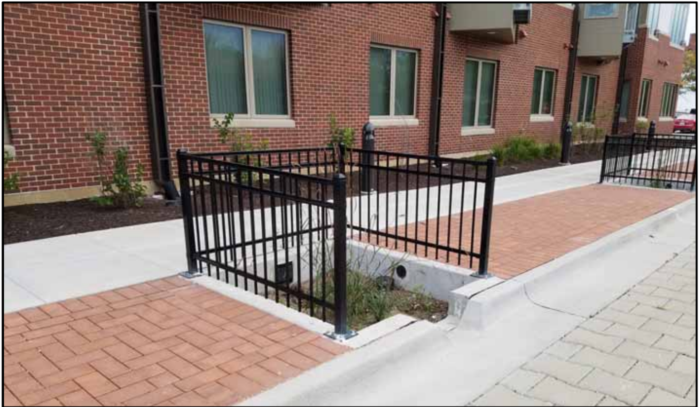
Figure 7. Tree well with Stormwater Management Feature
