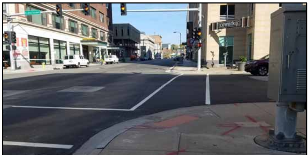
Figure 14. Misaligned Crosswalk due to Corner Ramp.
