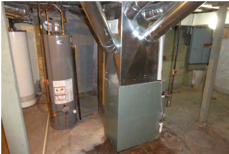
View of the furnace for the ground floor in the basement
